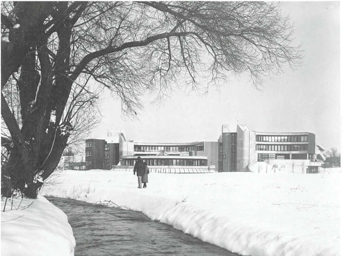
The new ESO headquarters building at Garching. Note that this picture was not taken on the day of the inauguration, but earlier in the winter.
