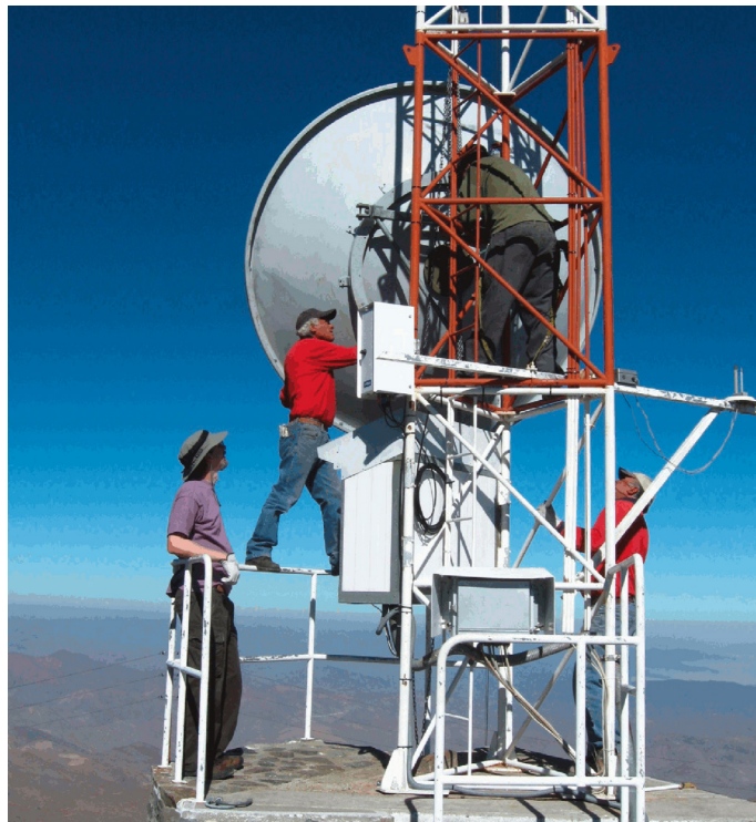
Figure 2. Installation of a 2-metre-diameter radio antenna on the La Silla weather tower. A matching antenna at Cerro Tololo receives the LSQ image data and transmits them to Yale over a high-speed internet link with the USA.
