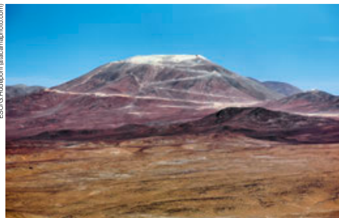
Rapid progress in flattening the peak of Cerro Armazones had been achieved by December 2014.
