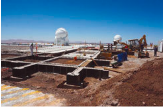
Construction work on the new AT station at Paranal.
