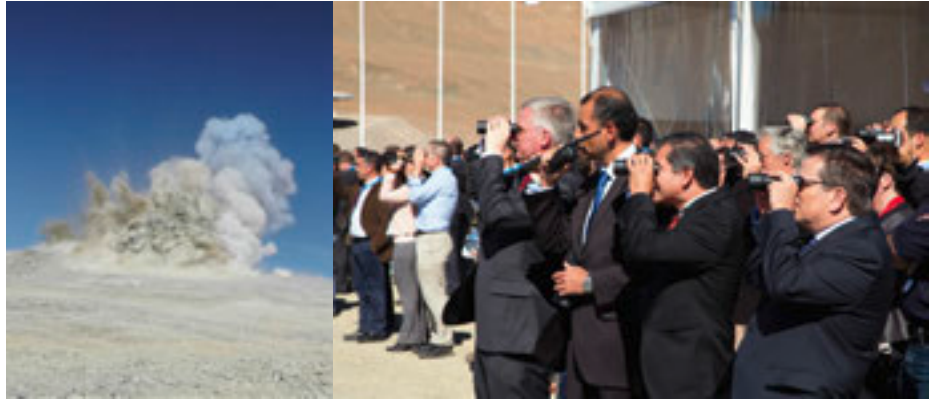
E-ELT groundbreaking event. Left: Part of the 3000-metre high peak of Cerro Armazones was blasted away as a step towards levelling the summit in preparation for the construction of the largest optical/infrared telescope in the world. Right (from left to right): ESO Director General Tim de Zeeuw, Chilean
