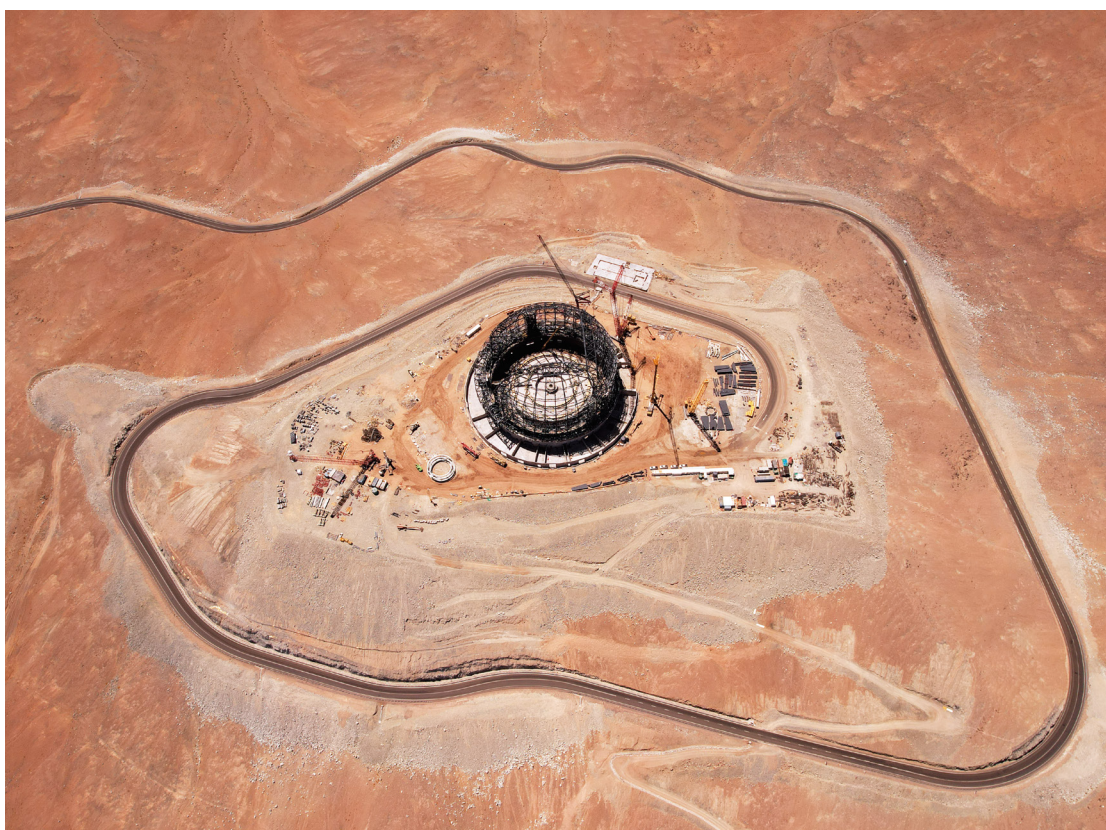
Aerial view of ELT construction on Cerro Armazones.
