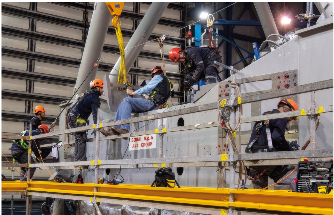
Upgrading the VLT Unit Telescope 2 centrepiece in preparation for GRAVITY+.
