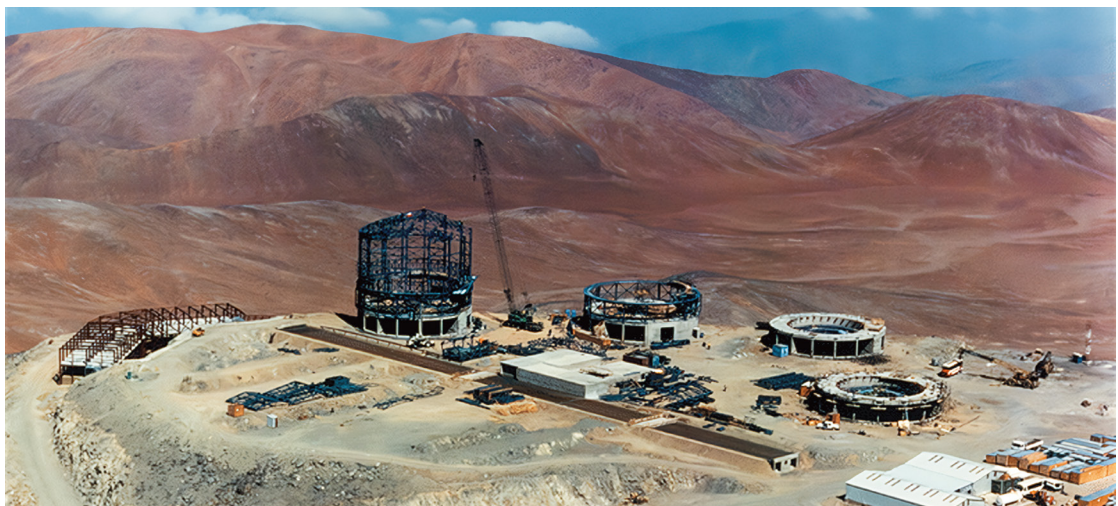
Top: The construction site of the VLT in 1996. Bottom: The VLT as it looks now.
