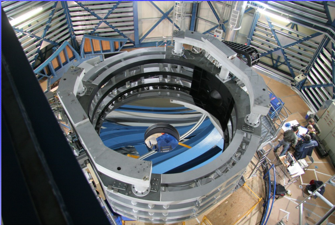
The VISTA Mirror Installed
