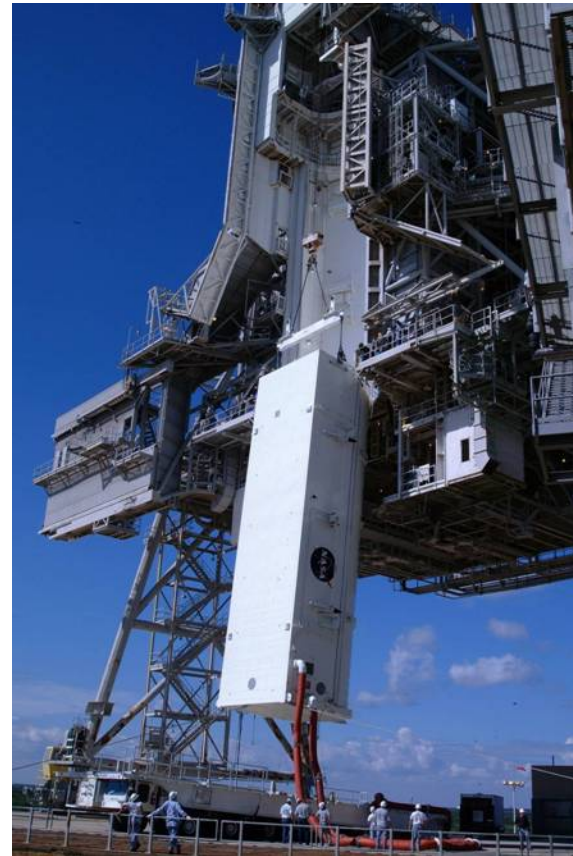
Canister Hoist at Pad
