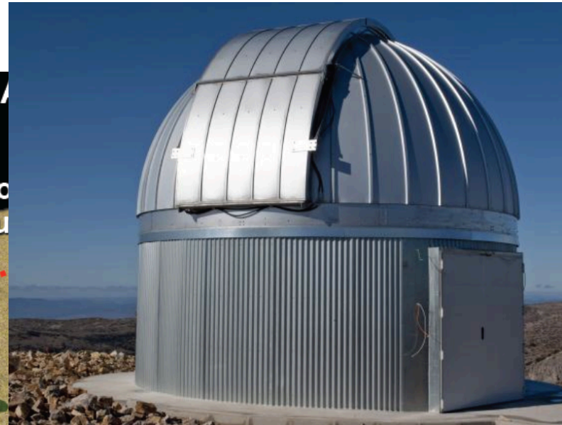
General Services Plant
