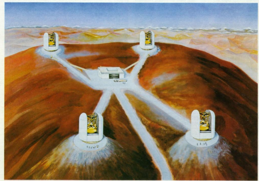
Artist's view of an early ESO VLT concept, representing a array of four 8 metre telescopes, of which two are shown to be linked for interferometric capabilities. It now seems preferable to do interferometry by adding to the large dishes a few smaller size (2–3 metre) telescopes that would be movable. (Drawing by J.-M. Leclercqz.)
