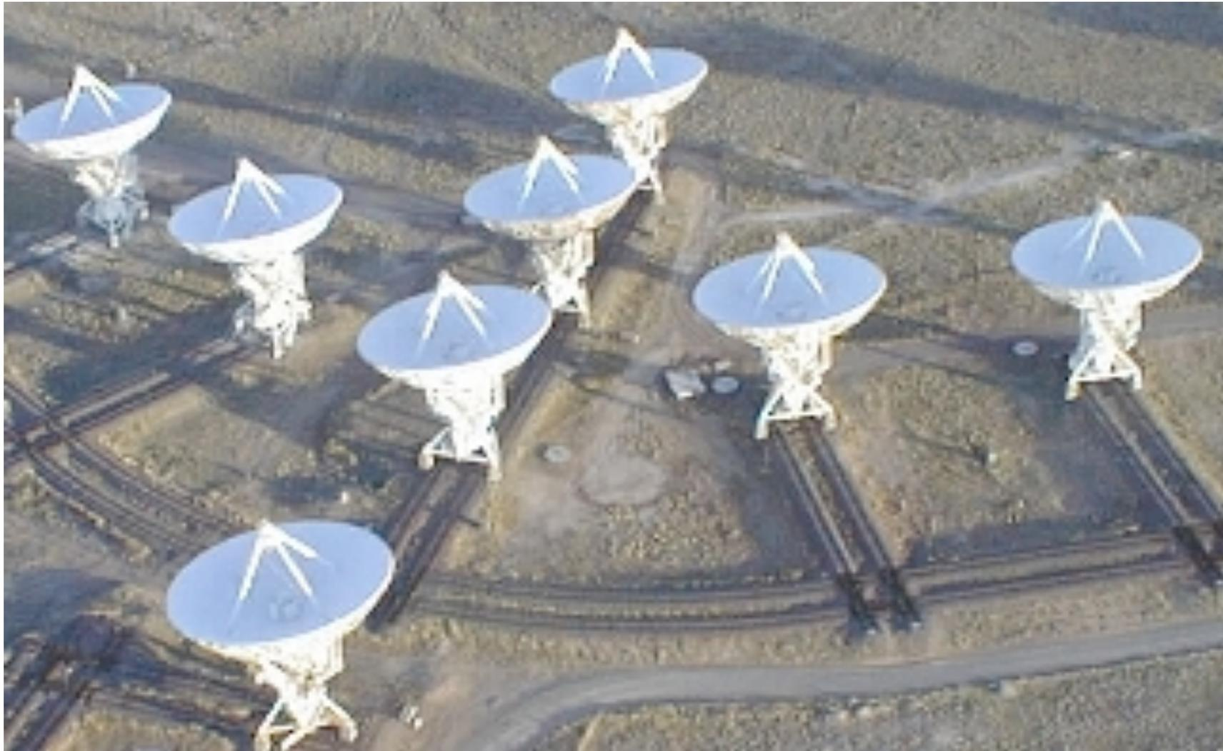
*The minimum spacing of the antennas determines the 'largest size of structure that can be measured'. Need a single dish measurement to obtain the total Flux Density*
