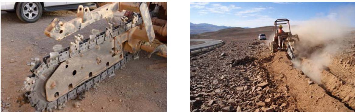
Figure 5. (Right) the cutting tool used to create the trench where the cable will be laid down and (left) the excavation.
