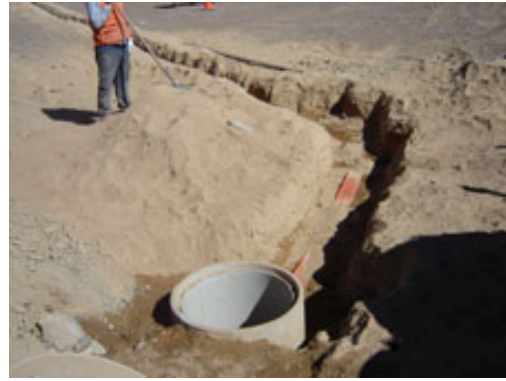
Figure 7. (Right) excavation for the installation of a concrete manhole (left) that will host the splicing box used to connect two consecutive sections of cable, about every 4km.
