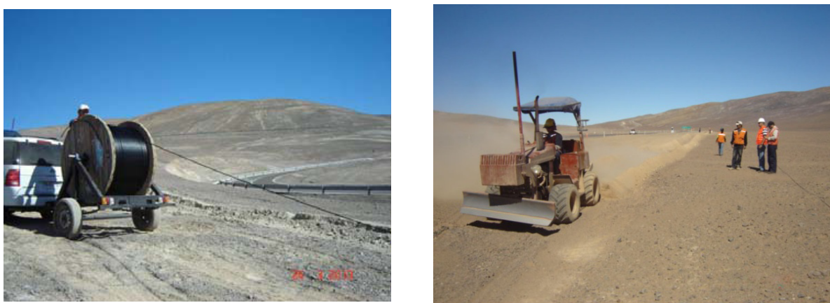
Figure 6. (Right) the fiber cable is directly installed in the trench that is then (left) filled back with excavation material that is then compacted.
