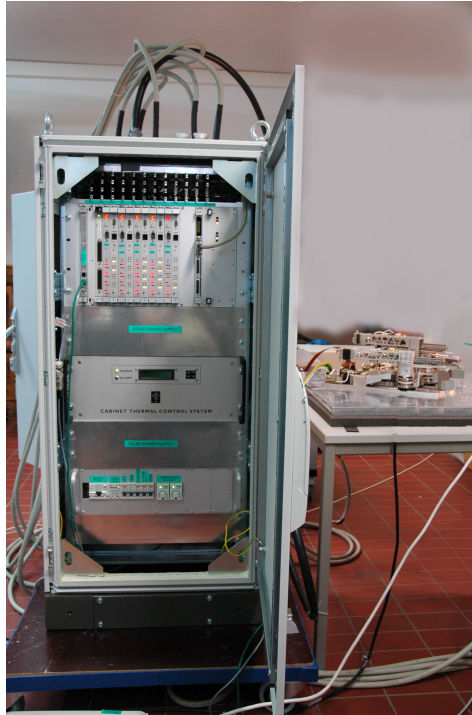
Figure 7: An advanced prototype of one of the final electronics cabinets controlling four of the KMOS pickoff arms during tests at USM.
