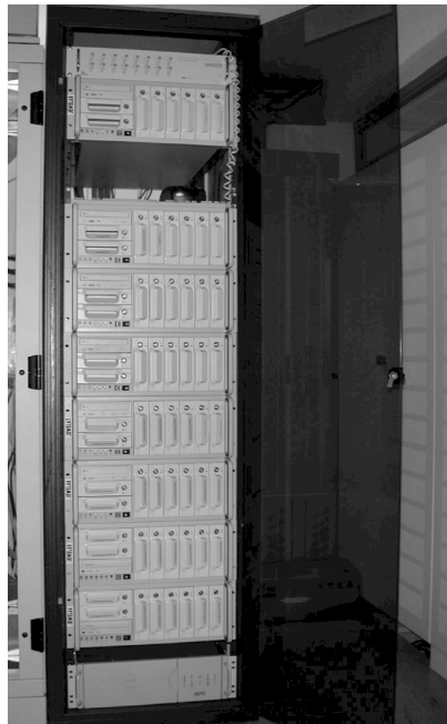
Fig. 2. This figure shows the first NGAS system in the Archive Operations Room in 2002. These servers were equipped with 8 times 80 GB disks each and had a total capacity of approximately 5 TB per rack. In addition, a sequential power on procedure has been put into place for maintenance reasons and to avoid overload due to starting current.
