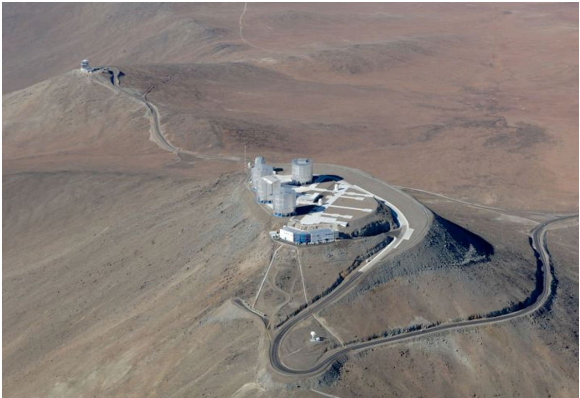
Fig 1. The ESO VLT on mount Paranal in northern Chile with its four 8.2m diameter Unit Telescopes, four 1.8m movable outriggers and VST 2.6m and VISTA 4m survey telescopes.
