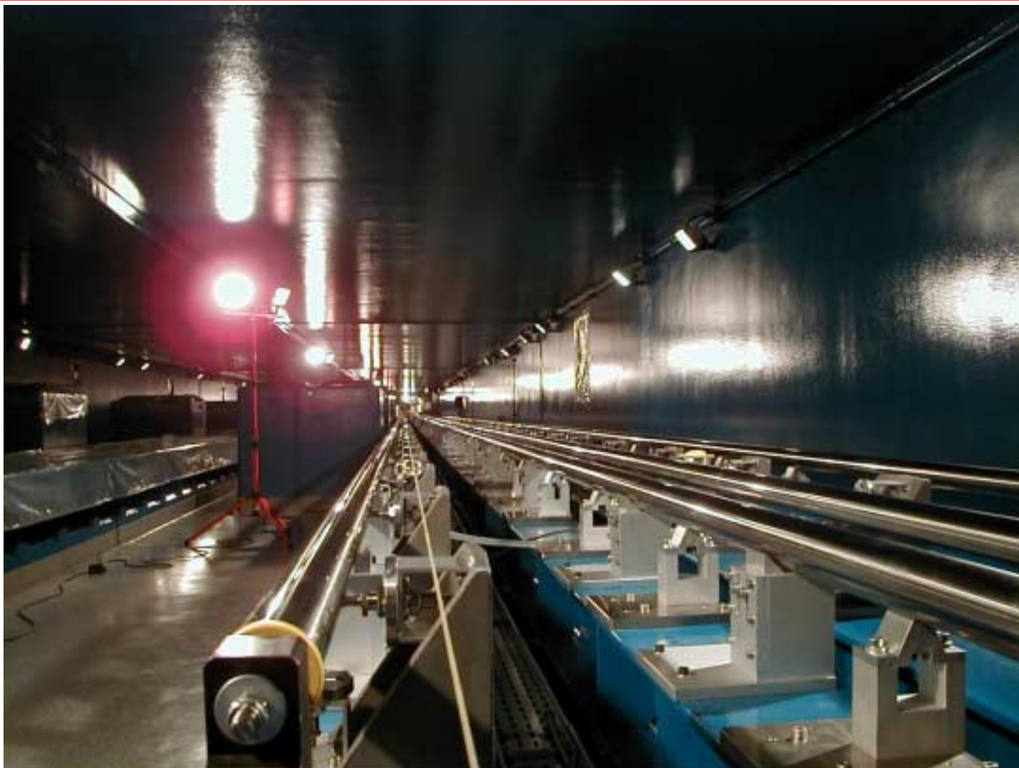
VLTI Delay Lines in the Interferometric Tunnel
