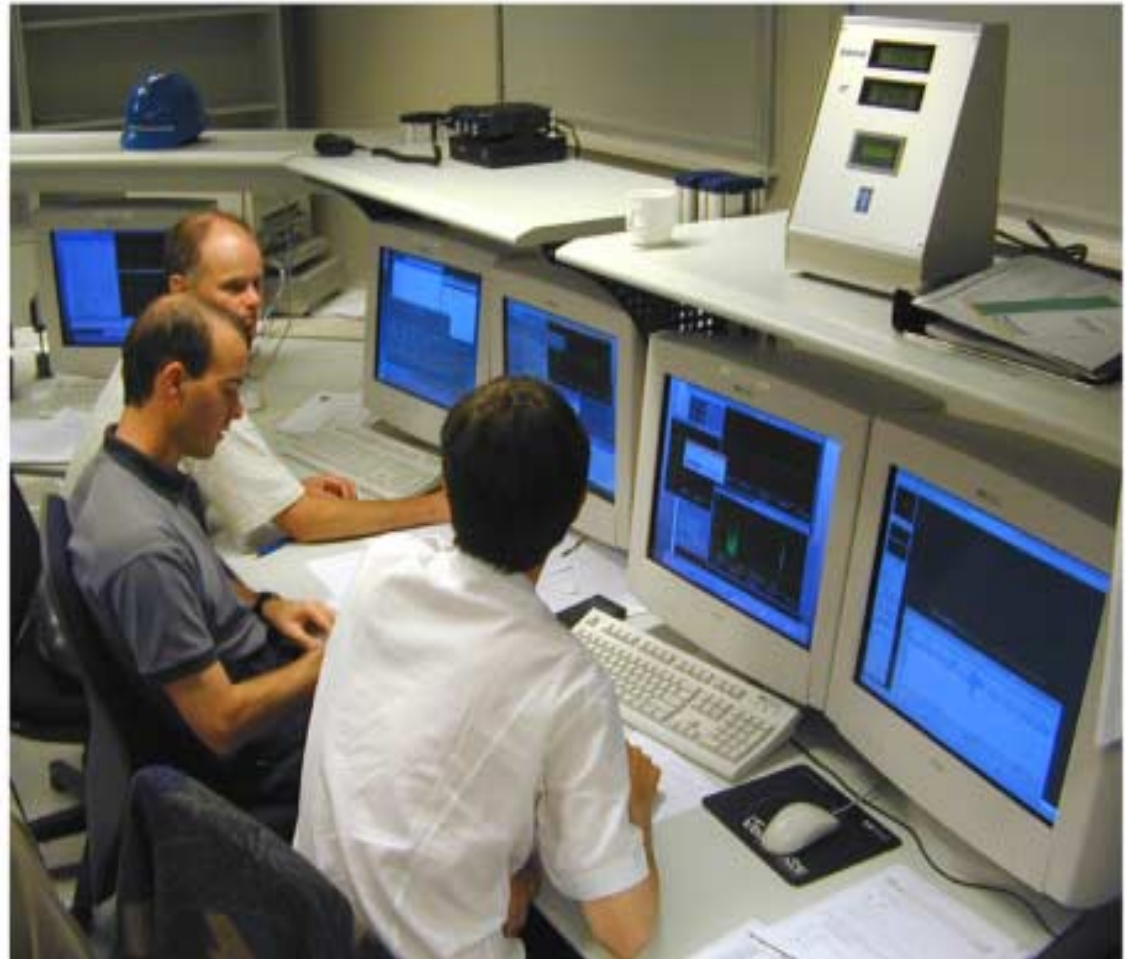
The VLT Control Consoles
