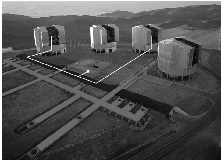
Fig. 5: Beam path followed by the laser beams during the test campaign at Paranal; it included all mirrors of the VLTI optical train up to the Nasmyth focus of UT1 and UT3. The maximum optical path length was 520 m (return way). The white circle indicates the location of the interferometric laboratory where the metrology beams were injected into the stellar paths.
