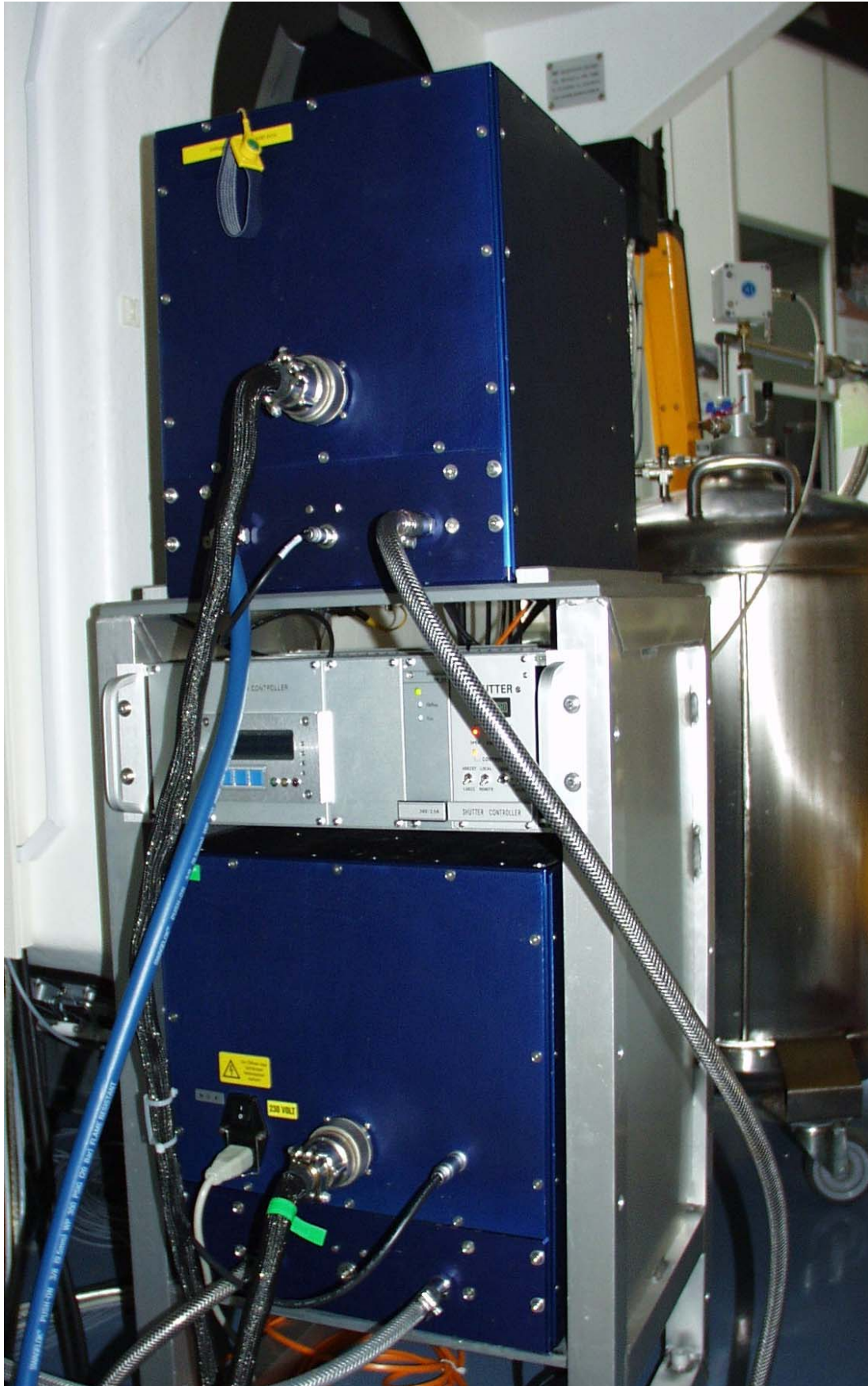
Figure 9.4-2, Power supply box, detector head box and PULPO+Shutter controller rack
