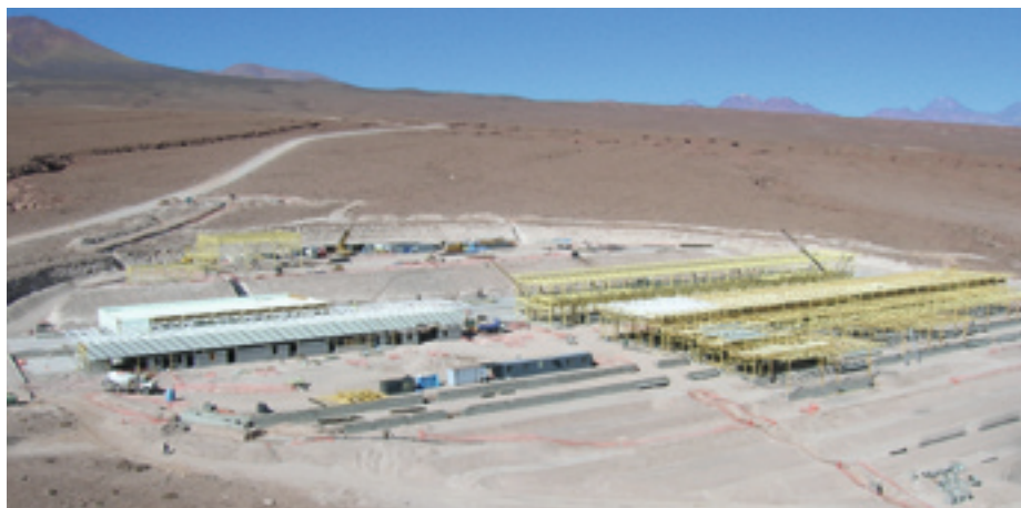
Figure 2: Construction work on the OSF Technical Buildings.
